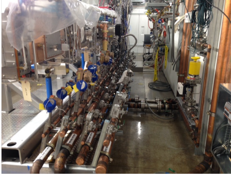
Figure 4.27: Distribution manifold for sending chilled water through the RFQ at multiple entry points (shown prior to final hosing installation.)
