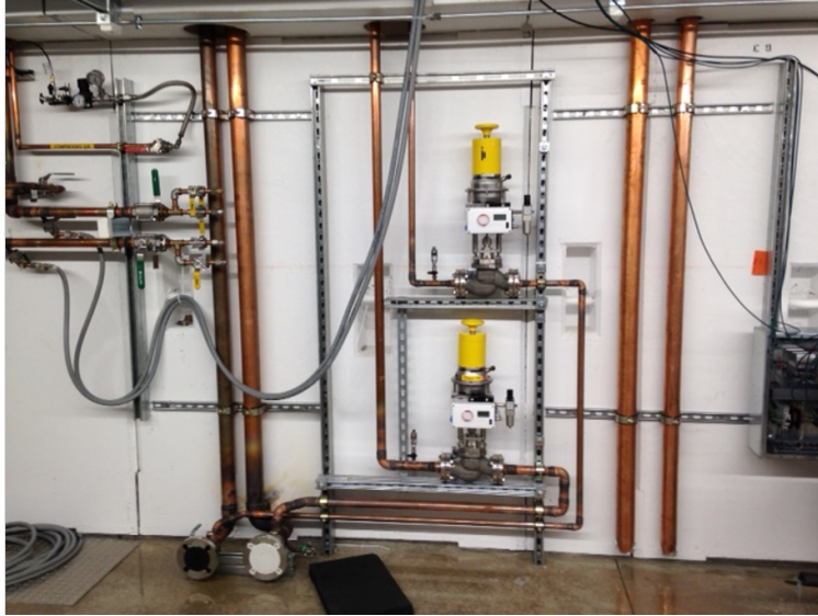
Figure 4.25: Flow valves for the wall and vane cooling circuits (yellow).
